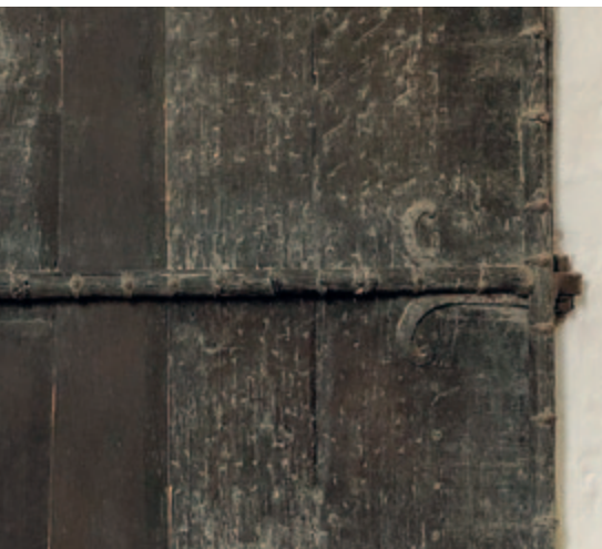
(32) Particolare della barra a Y con occhiello presso la chiesa di St Botolph ad Hadstock - Essex. Foto: www.rakinglight.co.uk . Detail of the Y-bar with eyelet at St Botolph's Church, Hadstock - Essex. Photo: www.rakinglight.co.uk .
